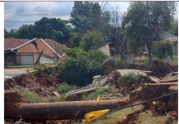
H12 pipeline exposure during December 2022
