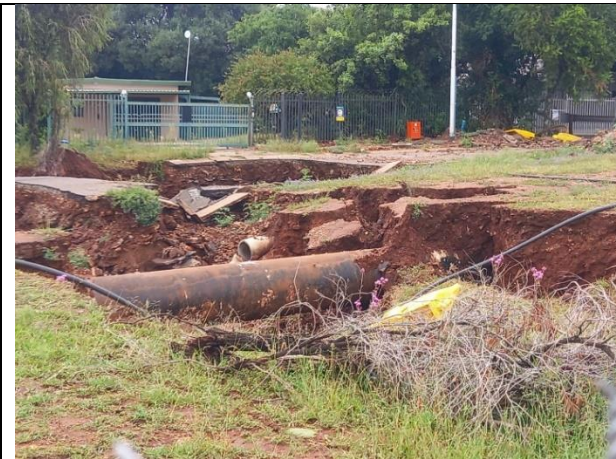
H12 pipeline exposure during December 2022
